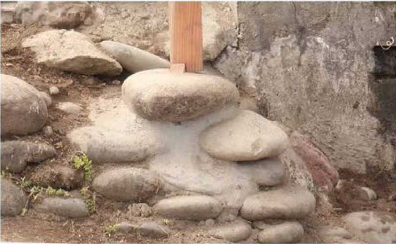
Dry-stacked stone and concrete-stabilized base, supporting timber post
