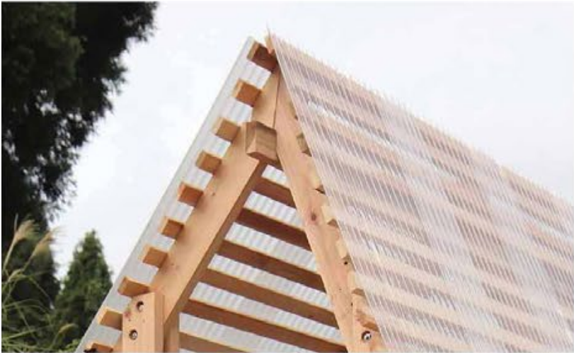
Exposed timber truss roof with a polycarbonate covering for diffused light filtration
