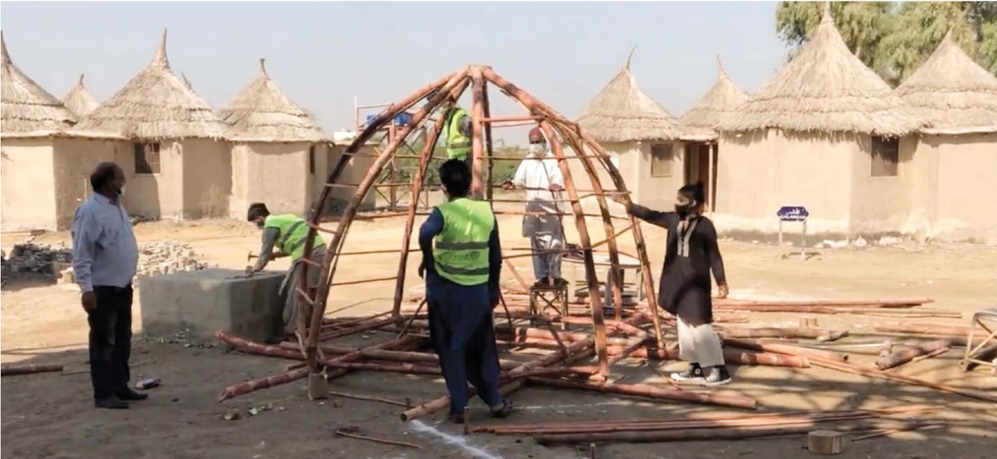
Bamboo pod typology constructed at Yasmeen Lari's 'Zero Carbon Centre Design Lab in Makli, Pakistan
