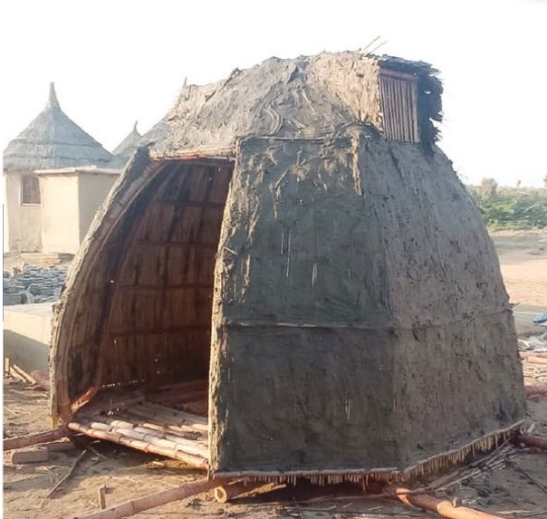
Bamboo pod clad with a thin layer of earth-lime plaster to provide shelter
